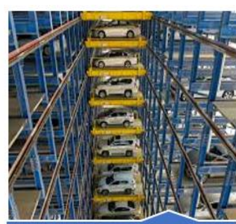
Robotic Parking System
