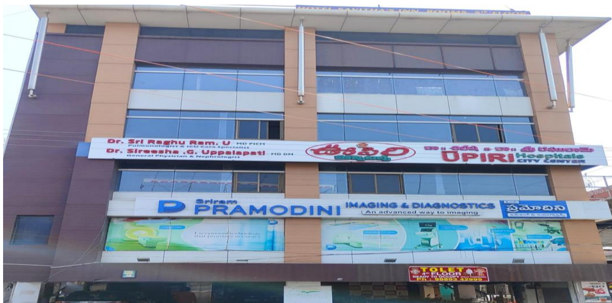
Branch office cum Diagnostic and Imaging Centre
